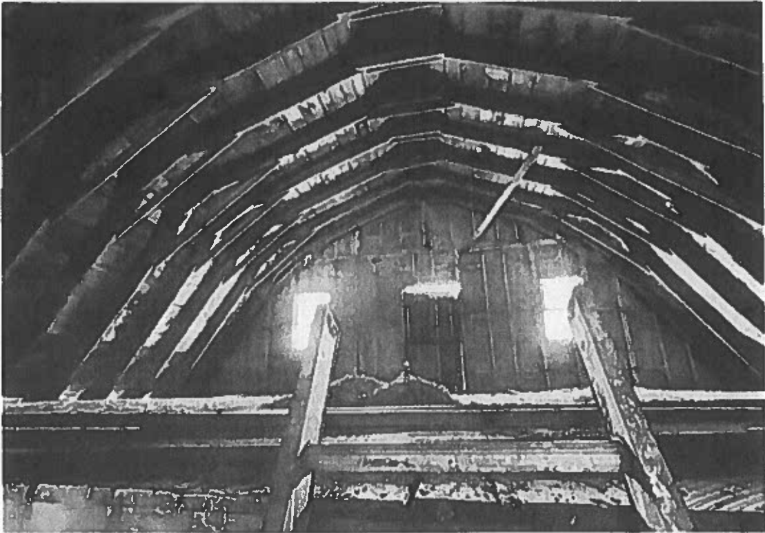
Additional Storage inside the Barn
