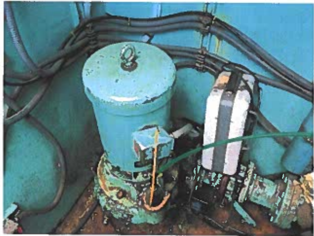
Existing Smith & Loveless Pump and Ancillary Equipment in Steel "Tin Can"
