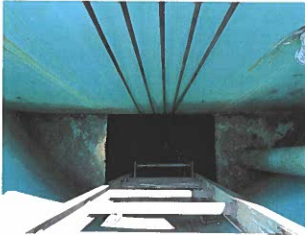
Existing Access (Manway) to Precast Concrete Wet Well
